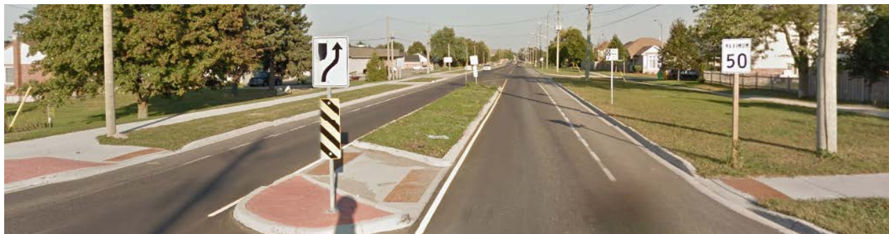
A pedestrian refuge island on Church Street, after the reconstruction
