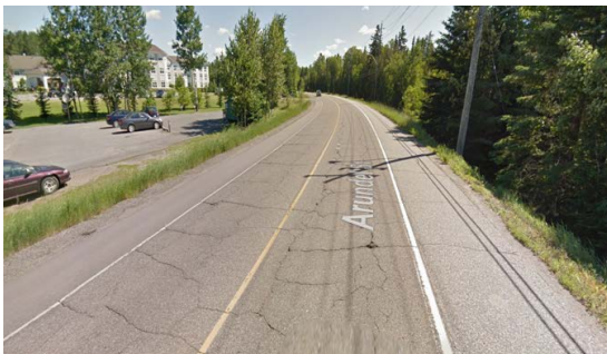
Arundel Street, before Complete Street transformation
