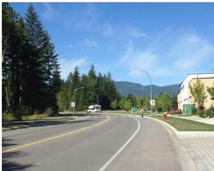
Murtle Crescent, developed according to the Road Cross-Section Bylaw, includes a sidewalk, bike lane, multi-use trail, lighting, a crosswalk, and street trees.
