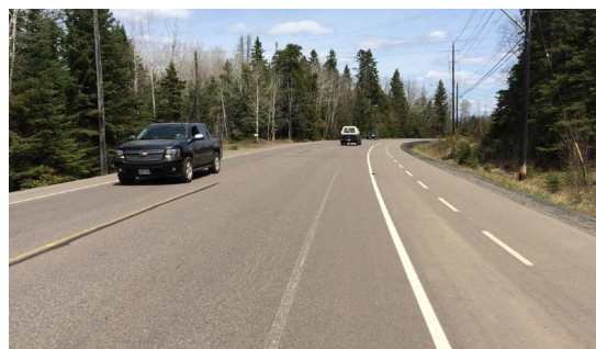
Arundel Street, south side bike lane faded, only one year after installation
