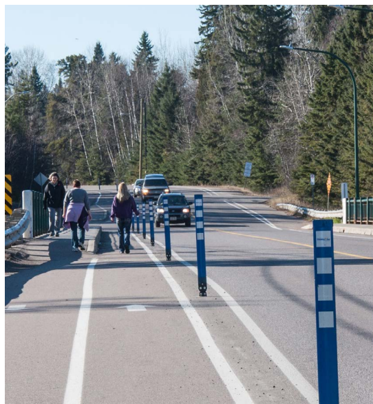
The modified design for Hudson Avenue, featuring an Active Living Corridor and painted buffers
