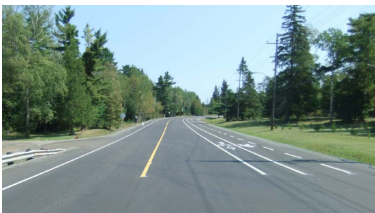
Arundel Street, with bike lanes on either side and a painted pedestrian shoulder
